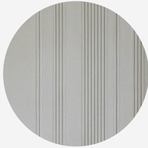
Accent wall Wall mouldings, installed vertically from floor to ceiling, painted to match the wall tone
